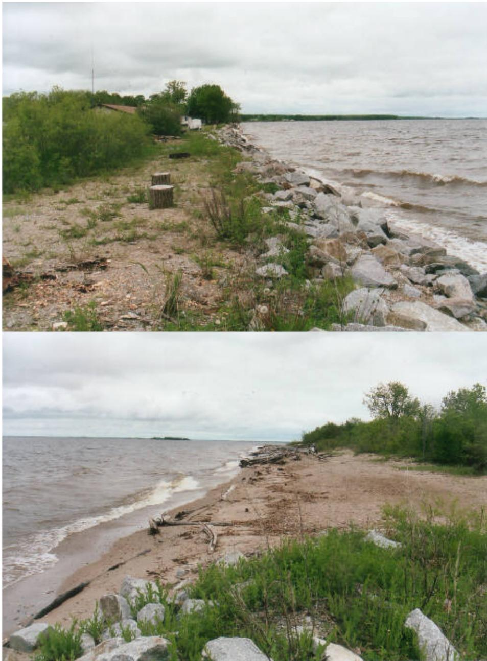
**Figure A1.1.** Photographs of the lake shore near Morris Point, 6/16/2004, showing sections protected with riprap (upper photo) and unprotected (lower photo).
